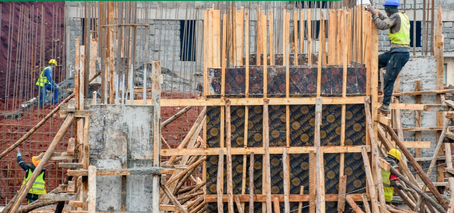
Ongoing construction works at a project site
