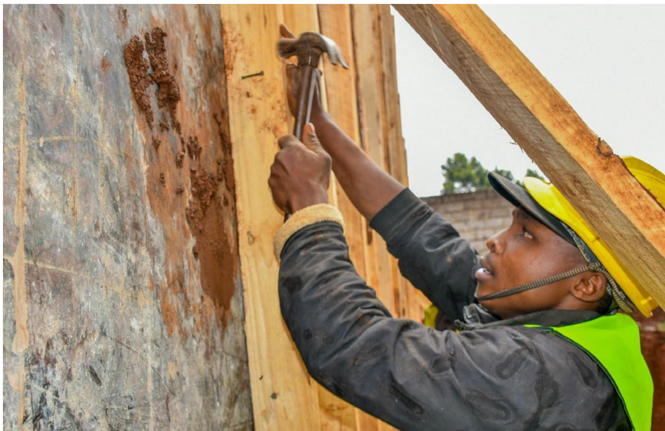
Paul Mwangi, a worker at Boma Yangu Kikuyu Affordable Housing Estate
