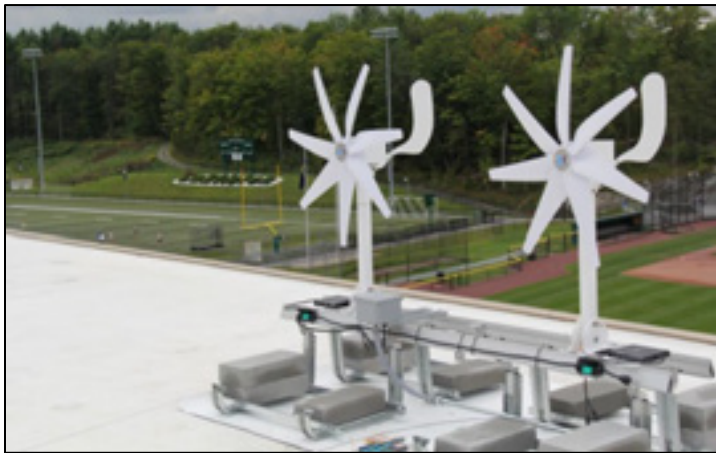
Figure 76: Rooftop wind turbines
