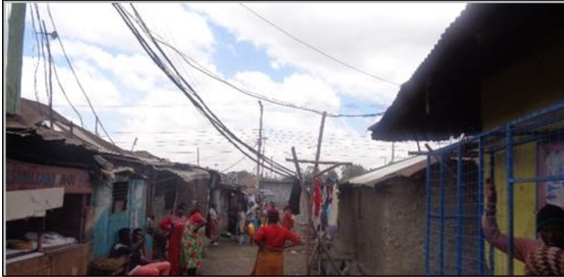
Figure 85: Unconventional Electrical Installations in Majengo
