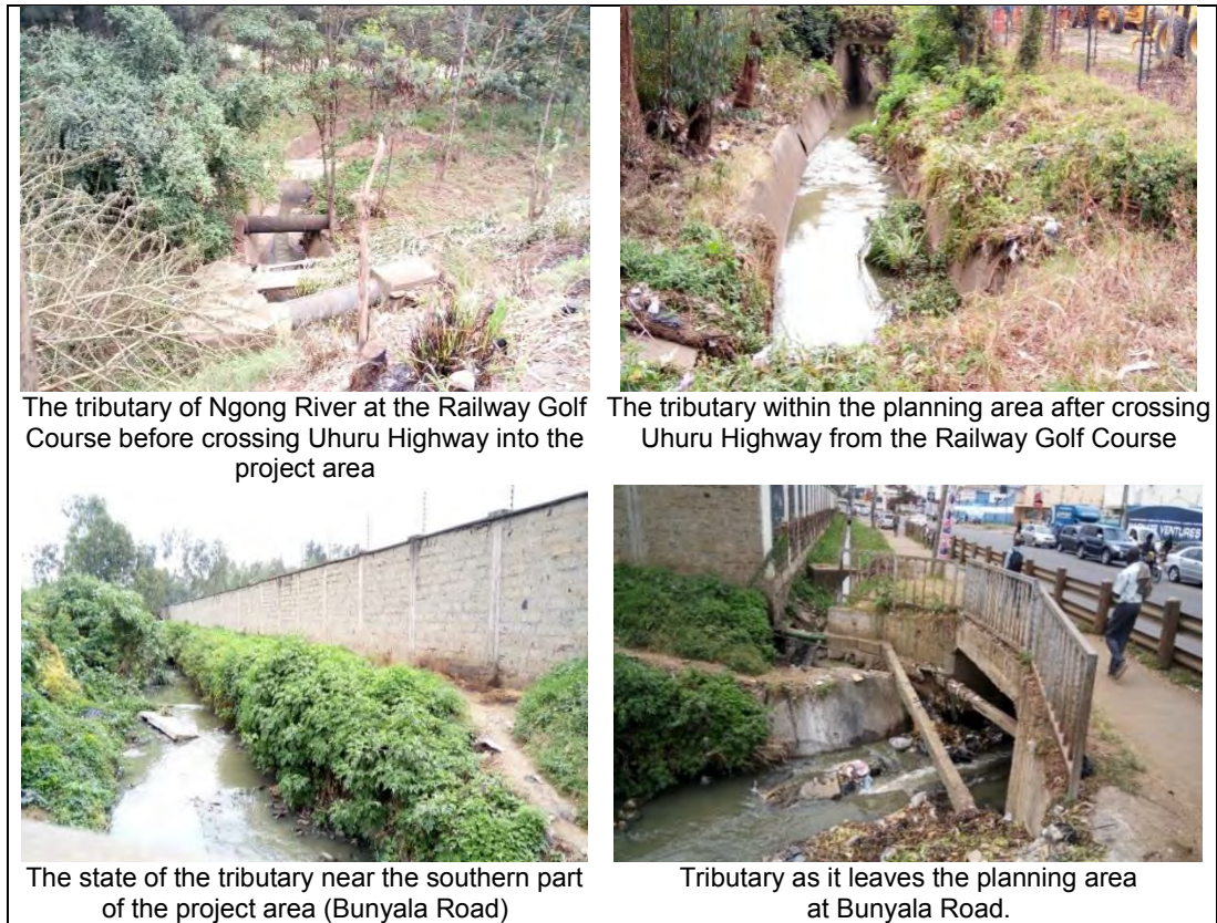
Figure 4-4 Ngong River Tributary Passing Through the Planning Area
