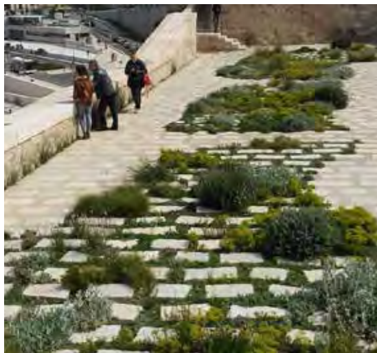
Vegetated cracks in paved surfaces path vegetation
