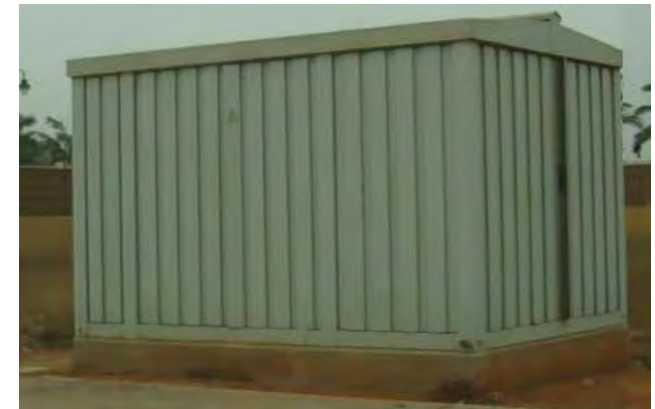
Figure 13.9: Typical Package Substation
